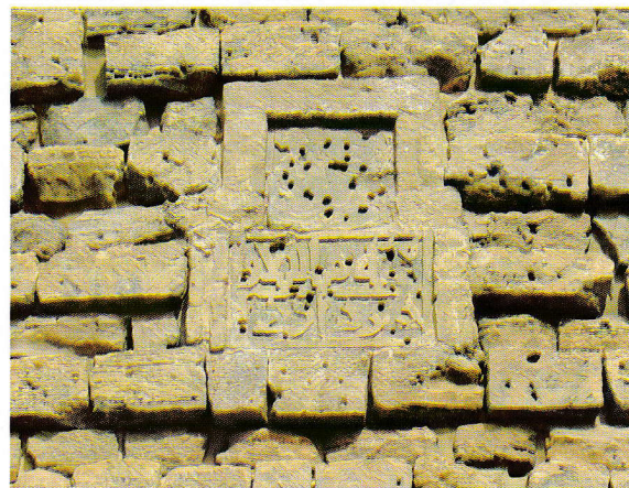
Inscription stone half way up on the south side, 60cm wide, 40cm high and 30cm deep. The Azerbaijani text in Arabic script reads "Davudun oğlu Mes'udun qüllesi" – "The Tower of Ma'sud, Son of Davud". The stone has been dated to the 11th century AD. It could be shown that the stone was placed during the construction of the outer wall. Photo: Erich Pummer.
