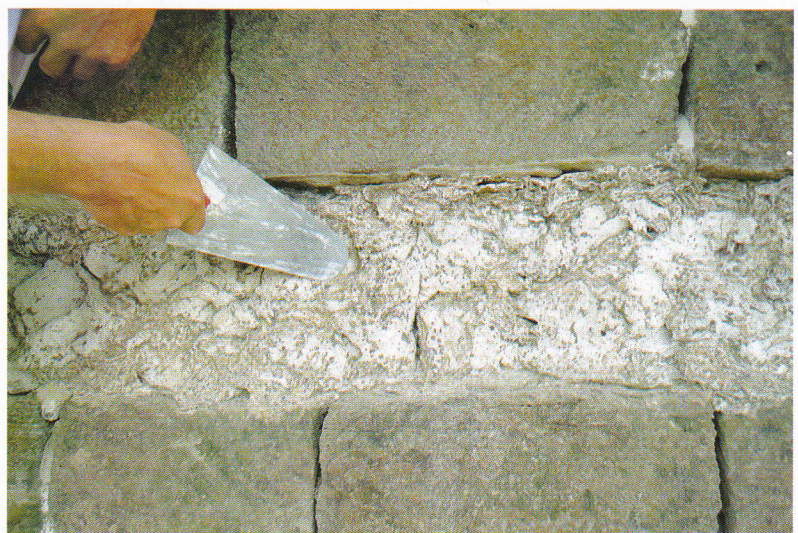
Mortar on the north facade of the tower. The imprint of mortar trowels and the method of working can be clearly seen here. Photo: Erich Pummer.
